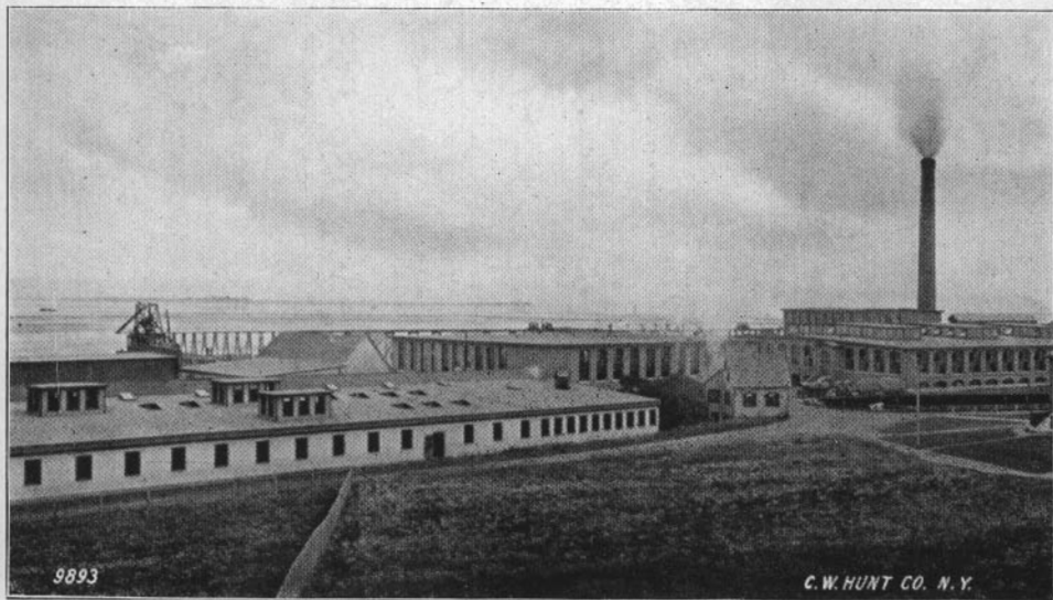
No. 9893. Cable Railway, Plymouth Cordage Co., Plymouth, Mass
