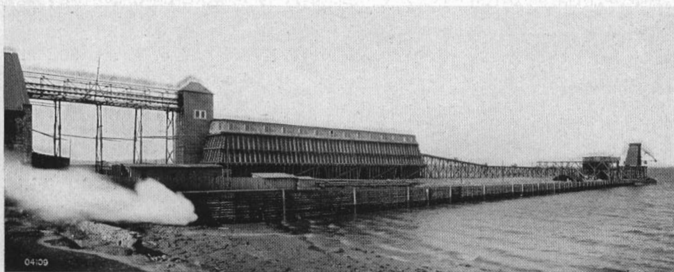
No. 04109. General View of the Cable Railway and Coal Handling Plant at the Fifty-second Street Power Station, Brooklyn Heights Railway Company, Brooklyn, N. Y. Track 800 feet long.
